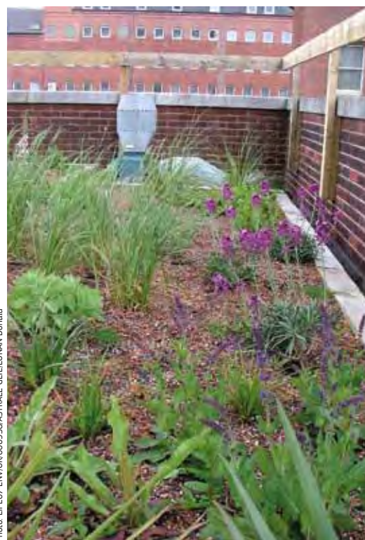
The GRACC project showed that green roofs reduce the heating and cooling needs of buildings
