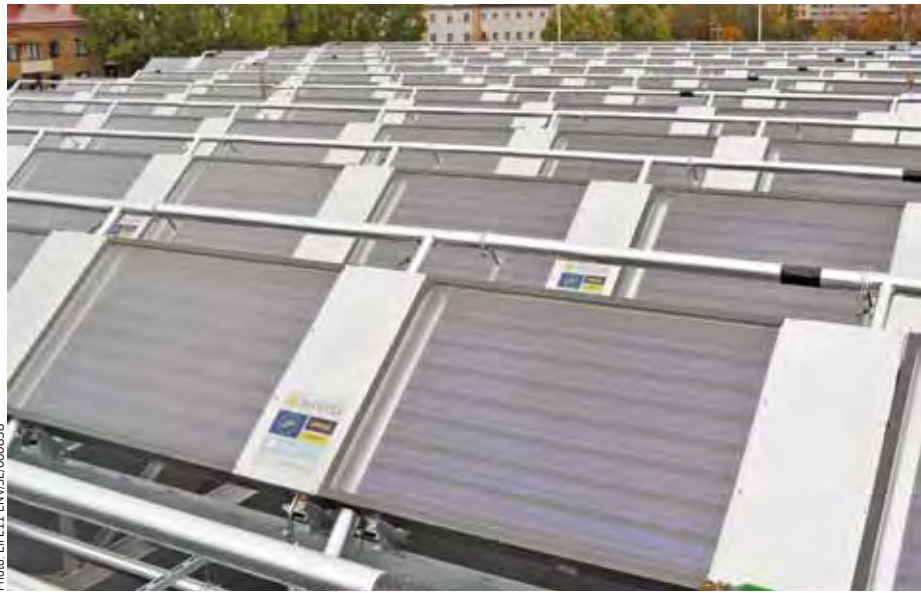
A Swedish project is testing the use of solar thermal collectors with a zero electricity heat pump and energy storage for sustainable heating and cooling
